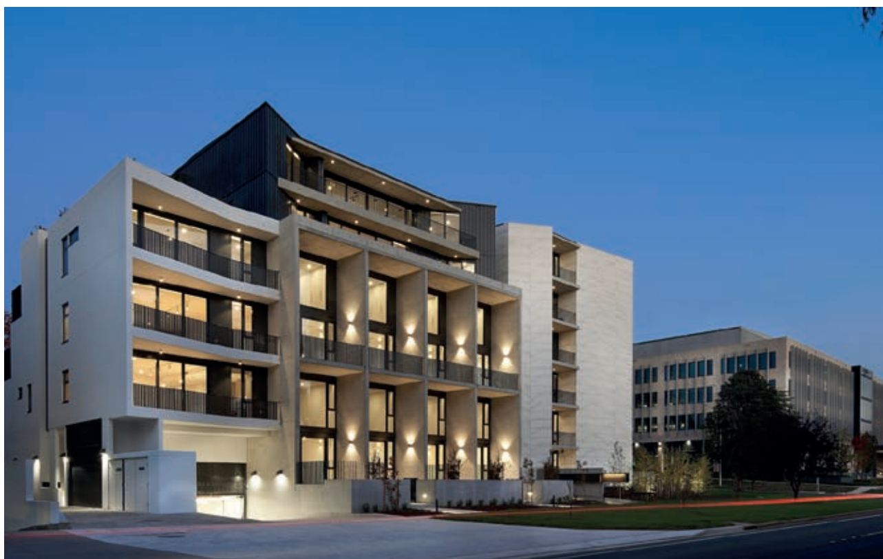
Dominion Apartments – Rooftop, terrazze e aree esterne Canberra, Australia Pedestal System – New Maxi NM
